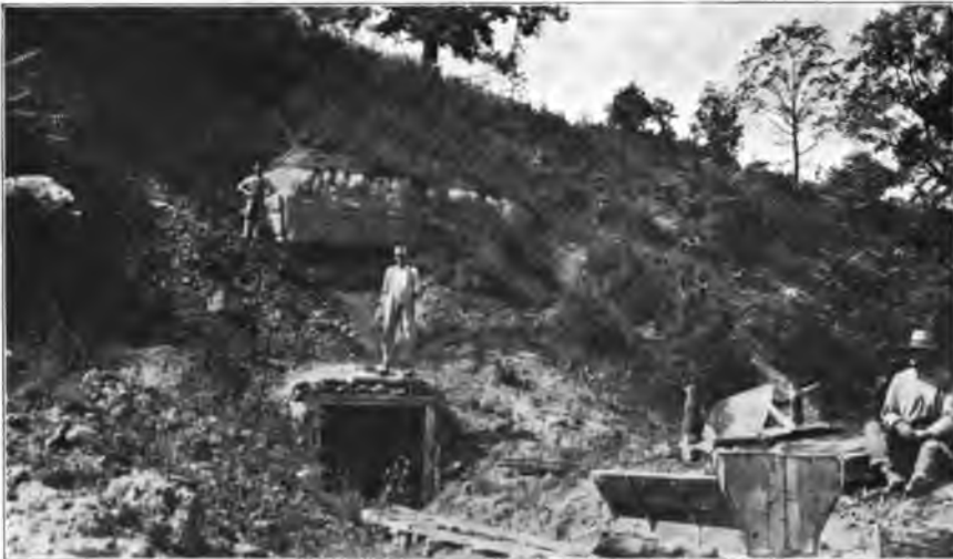
B—The Carl Crabtree mine in which Tionesta clay is mined for the general market. Putnam Hill limestone exposed about 15 feet above the mine. Blunt Run, Muskingum County (Locality 27)
